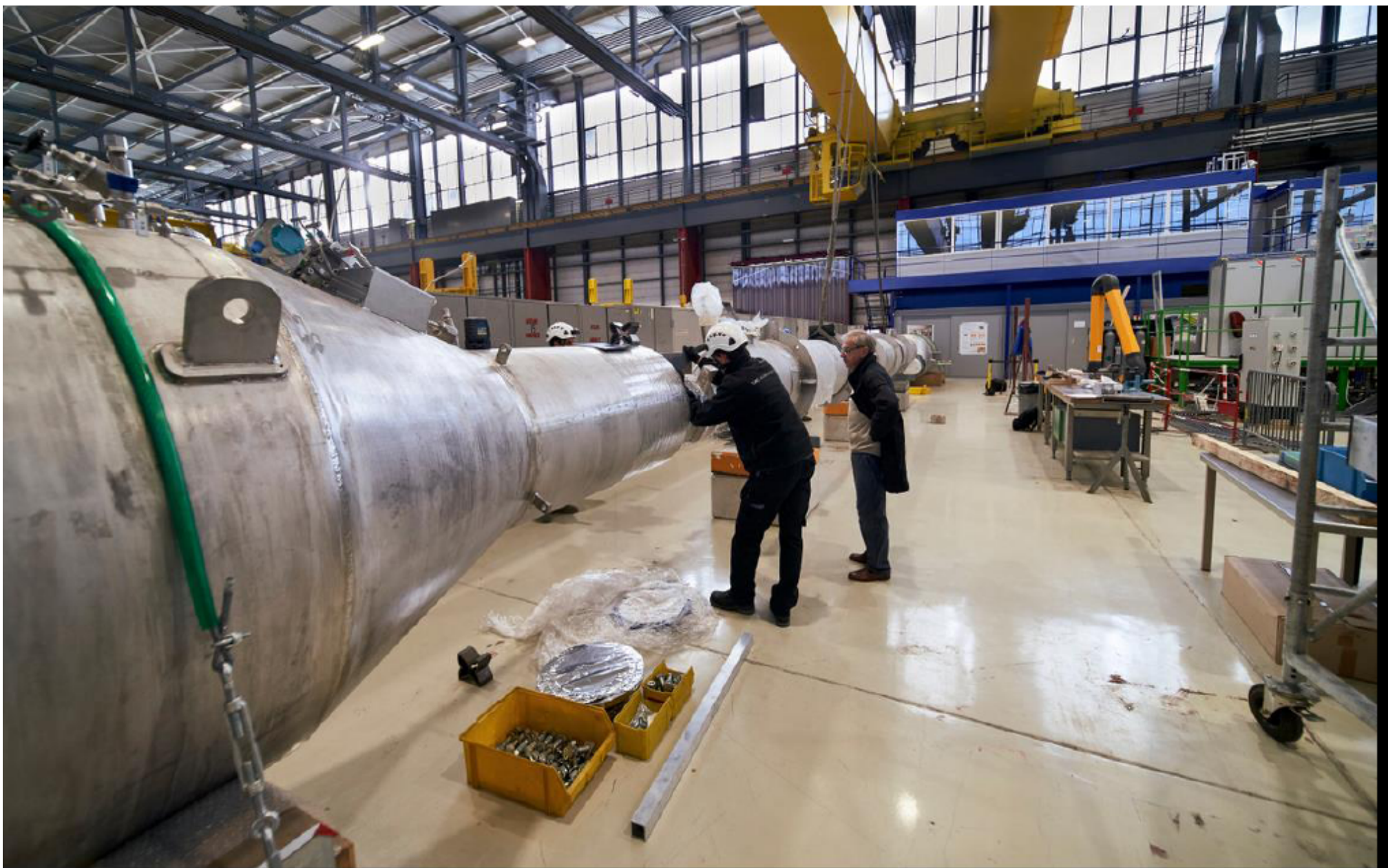
On Friday, 24 November, ARIA's top and bottom modules plus one standard module were brought to Building 180 and lined up to precisely test their alignment and interconnections. (Image: Max Brice/CERN)
