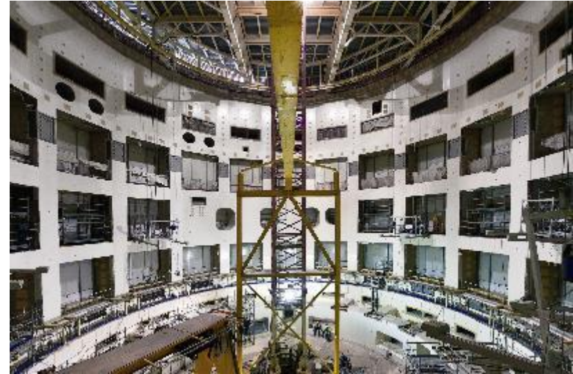
Tokamak assembly pit (Ferrovia)
