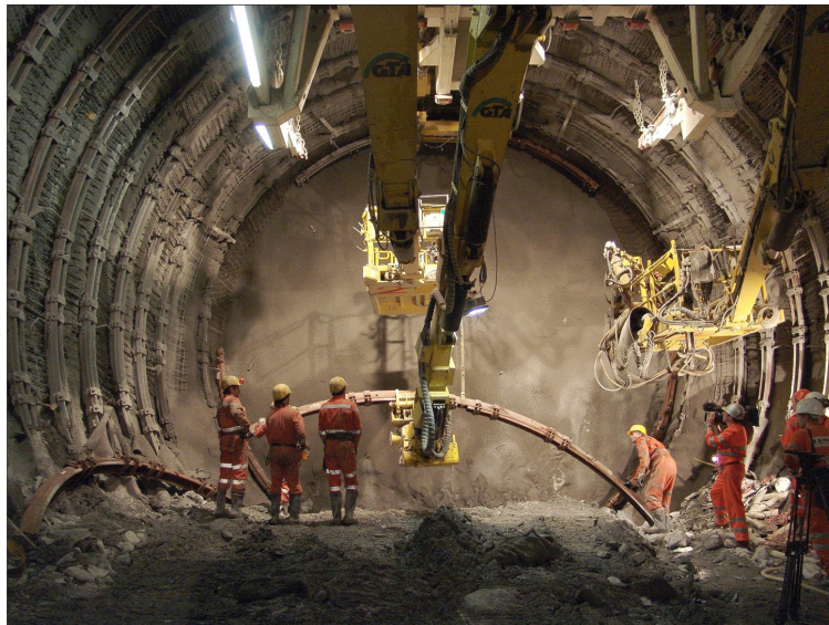
Figure 81: Support of the tunnel walls can be erected in parallel to the drilling process.
