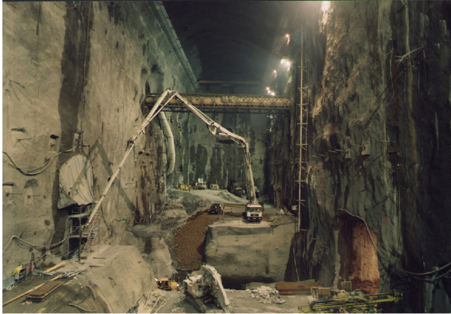
Figure 75: The construction of the Robert Bourassa hydropower station in Quebec, Canada. Drill and blast was used to excavate the powerhouse with dimensions 296 m by 25 m by 47 m. More than 11,000 rock bolts were used.
