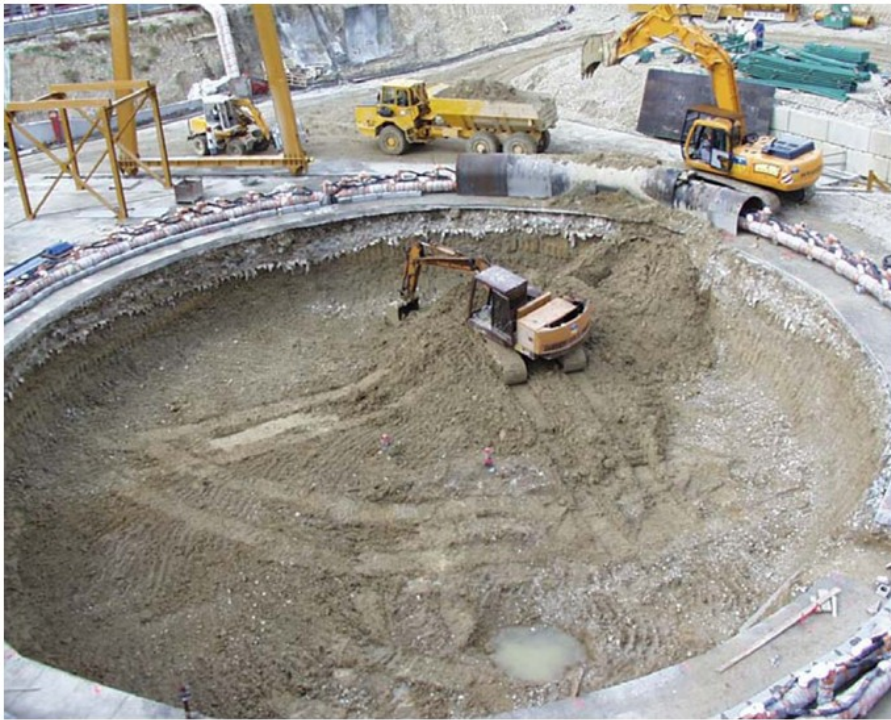
Figure 86: The construction of the CMS access shaft for the LHC project at CERN, Geneva. This shaft has an 18 m diameter and the entire CMS experiment was lowered through it. To facility its construction, the ground at the shaft walls was frozen.
