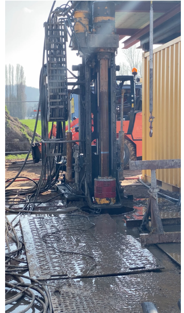
Hombourg, Sint Pieters Voeren and Gemmenich drilling completed on schedule
