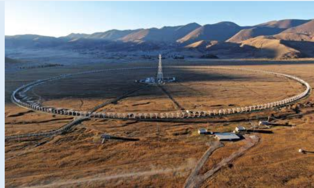
The 313-unit full system of the circular array solar radio imaging telescope
