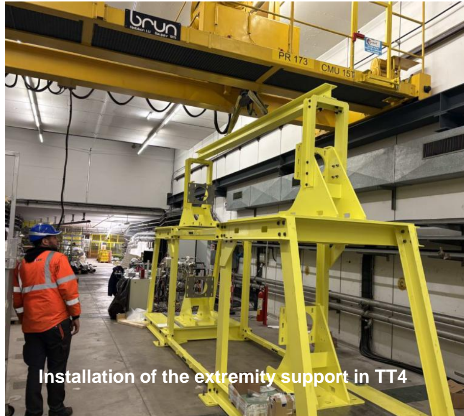
Test of support installation and alignment in TT4
